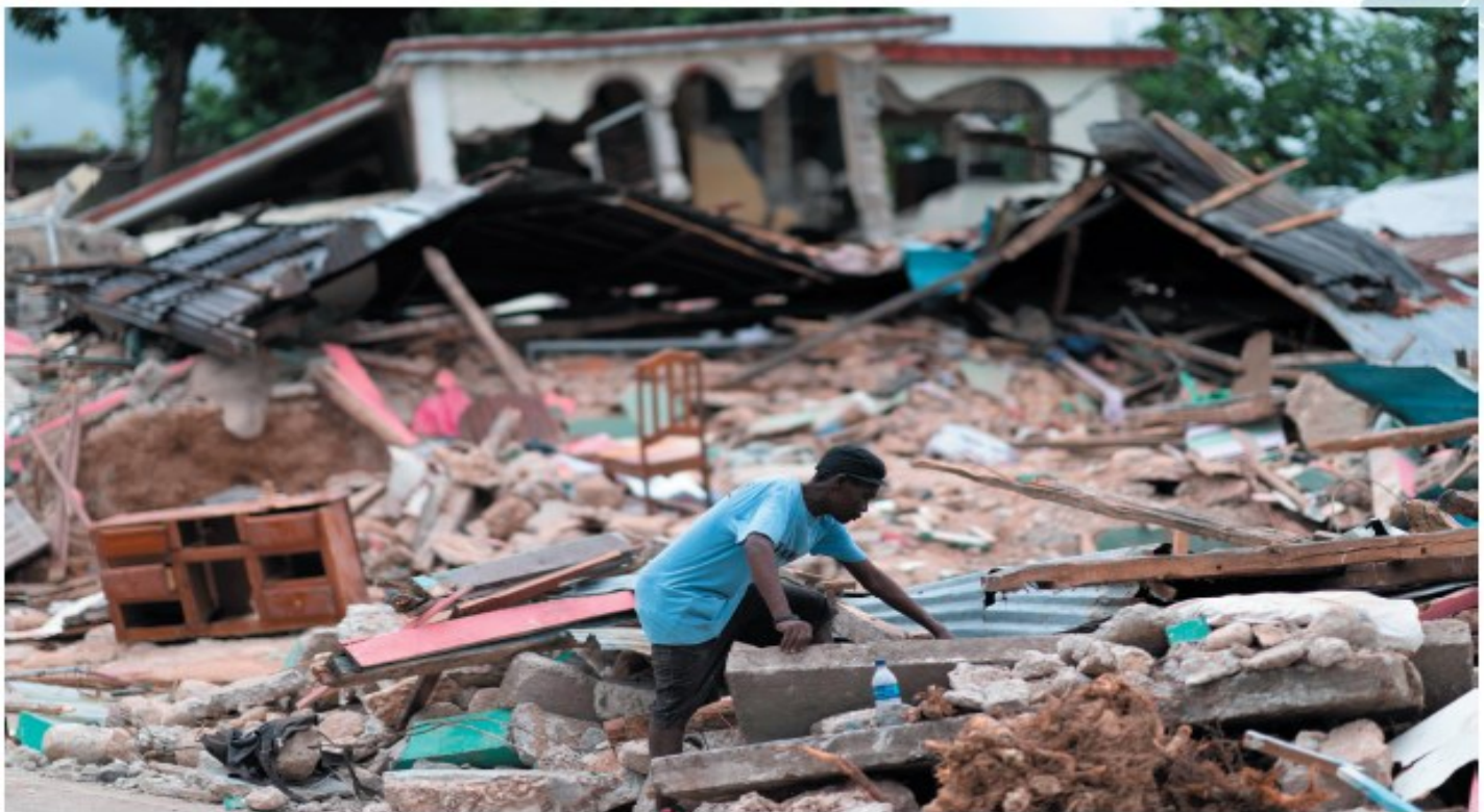
A man searches the debris of a collapsed house in Les Cayes, Haiti, after the earthquake. Photo by David de la Paz/Xinhua/Alamy Live News
